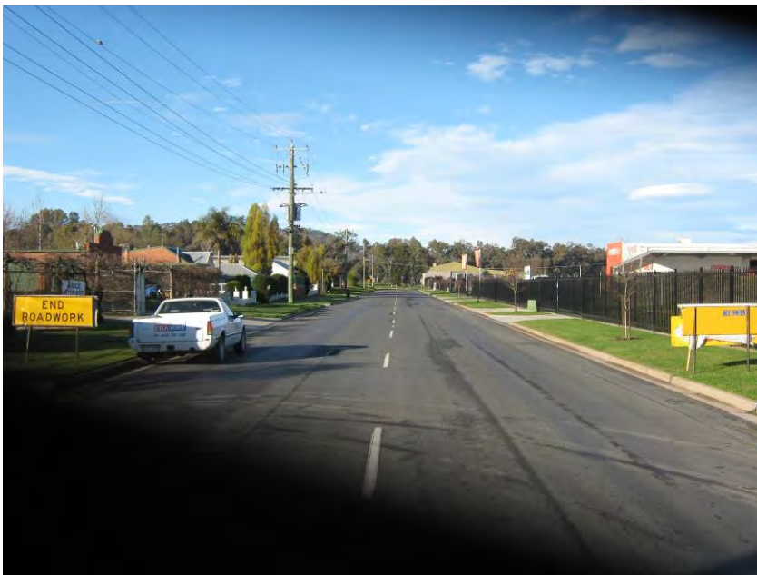
Figure 6 Schubach St: approx 200m looking south to the intersection
