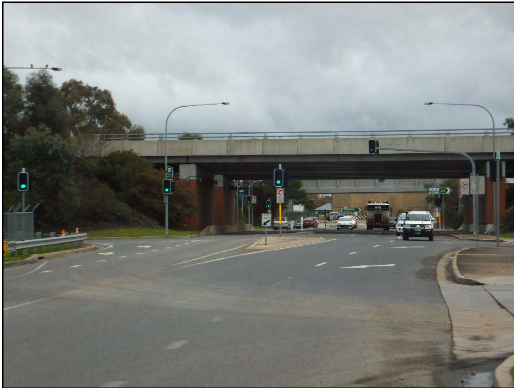
Photo 2 looking west along East Street approaching East Street/ Hume Freeway Interchange
