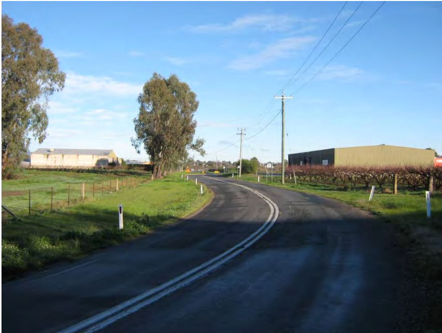
Figure 1 Doctors Point Road:- approx 180m east of the intersection
