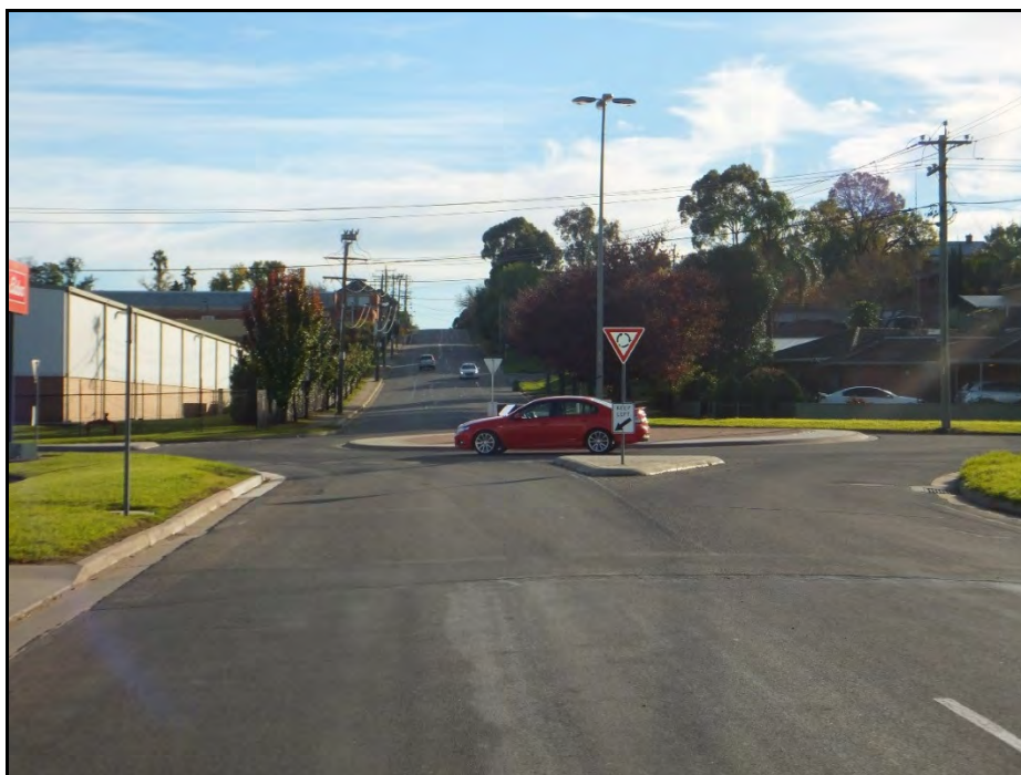
Photo 1 looking north along Schubach Street approaching roundabout
