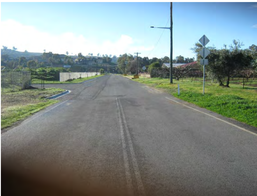
Figure 2 Willowbank Road:- approx 250m west of the intersection
